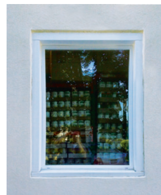
The before and after conditions of the building.
